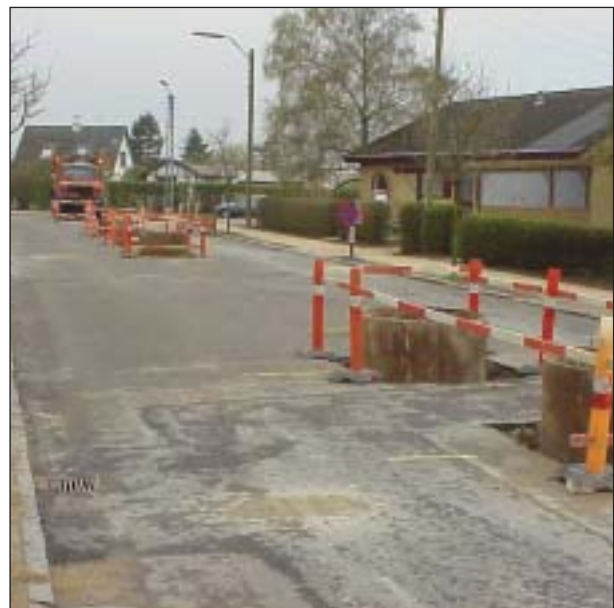
Vertical supports positioned above lateral connections.
