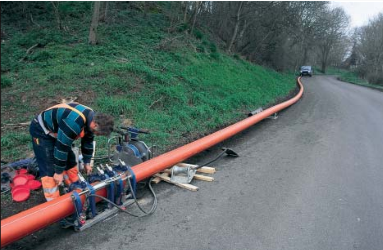
PE pipes are fusion-joined prior to installation.
