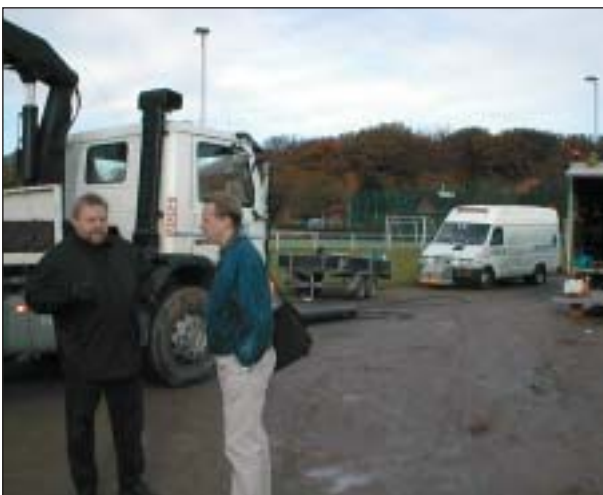
The control committee inspects work site layout.
