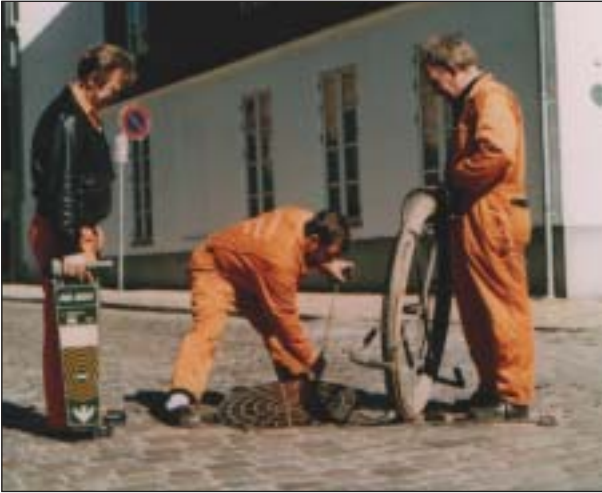
Operators carrying out inspection.
