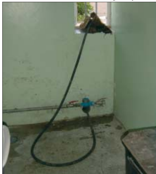
Pre-bored hole in basement for inserting an impact mole.
