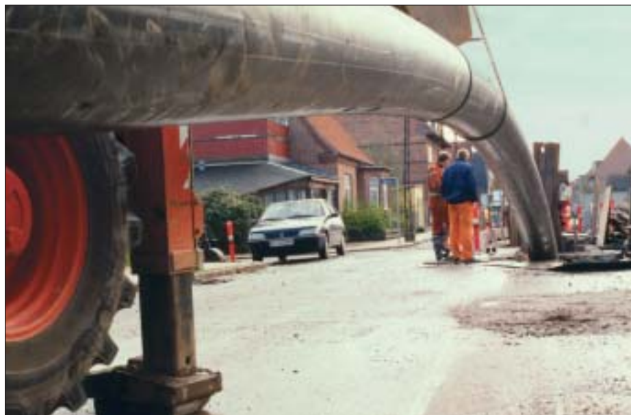
Sliplining work site.
