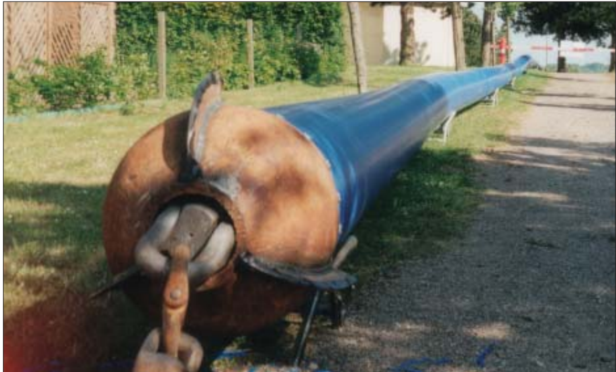
Fuse-joined PE pipe ready for installation.
