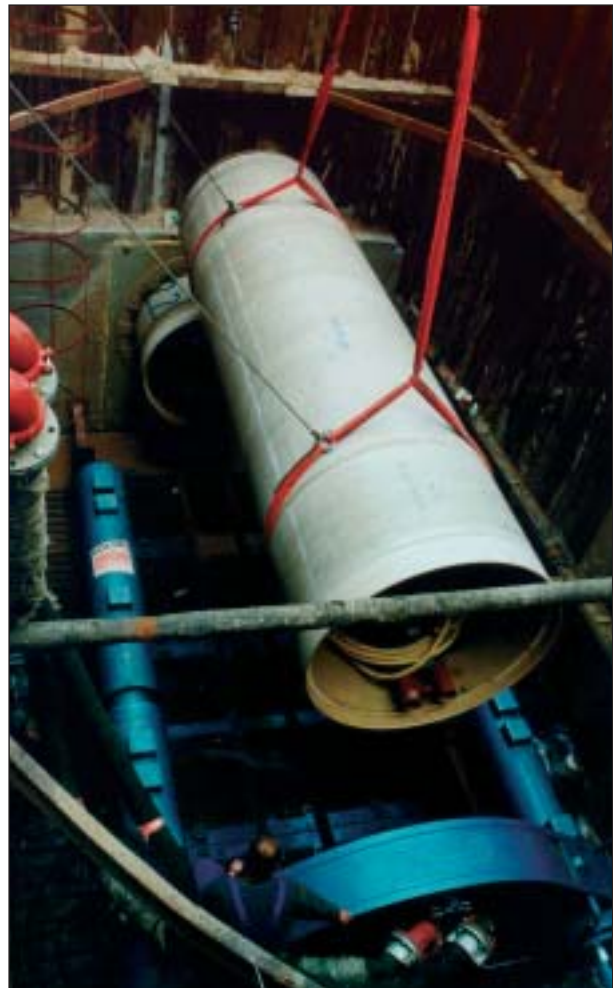
Microtunnelling launch pit. Jacking a fibreglass pipe.
