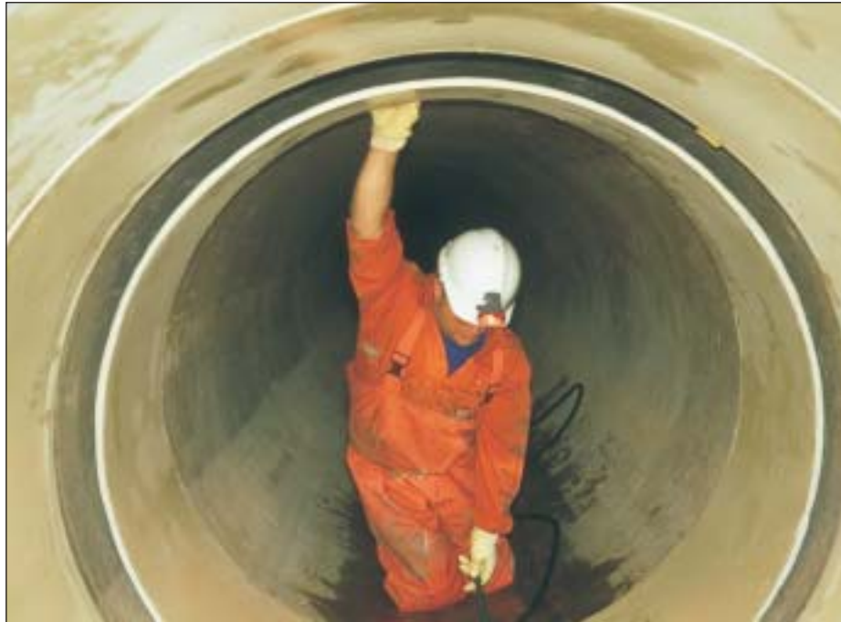
Fitting panels in an existing pipeline.
