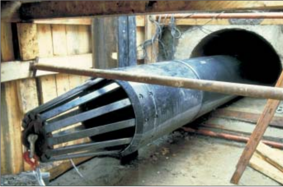
Preparing to pull in a 500 mm diameter PE slipliner.
