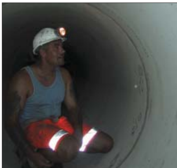
Checking the installation work.
