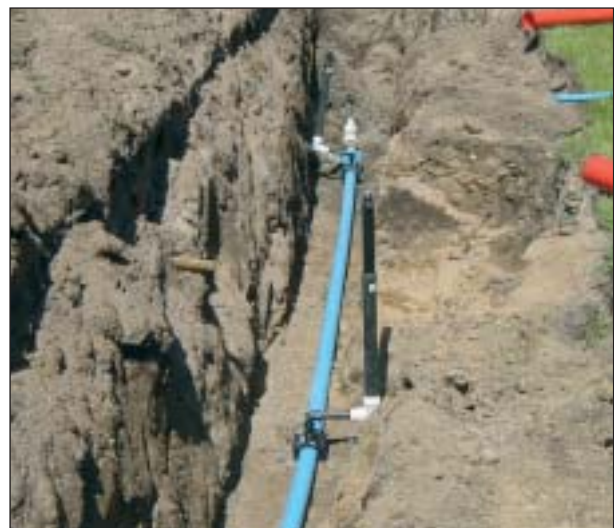
Renovating water pipes in a residential area.
