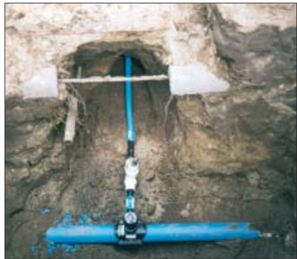
Renovating water pipes close to the foundations of a building
