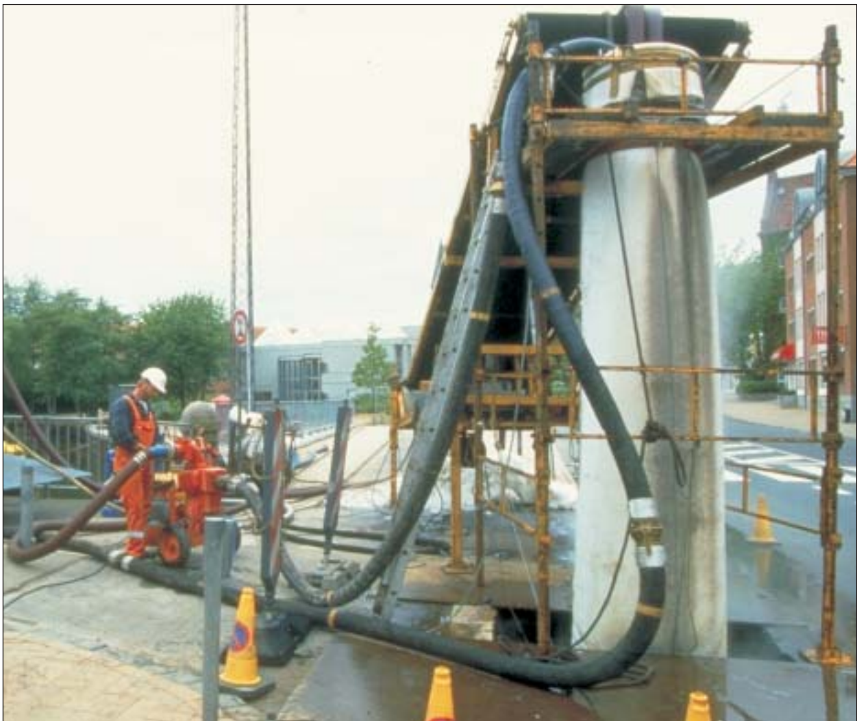
Cured-in-place lining
