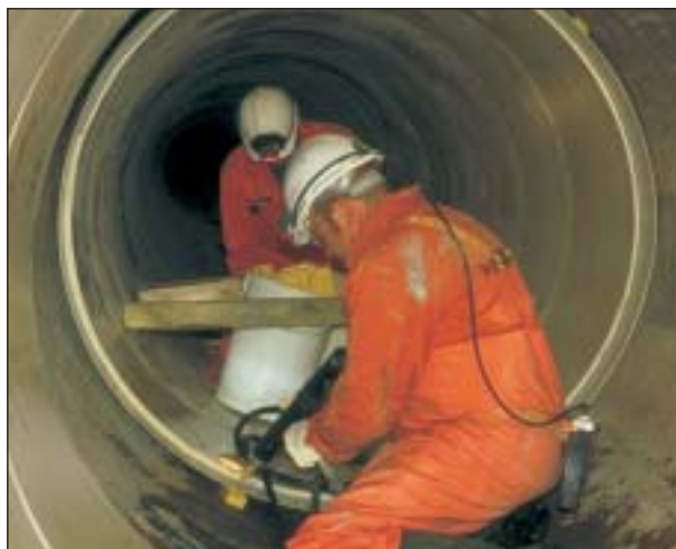
Fastening panels to the existing pipeline.
