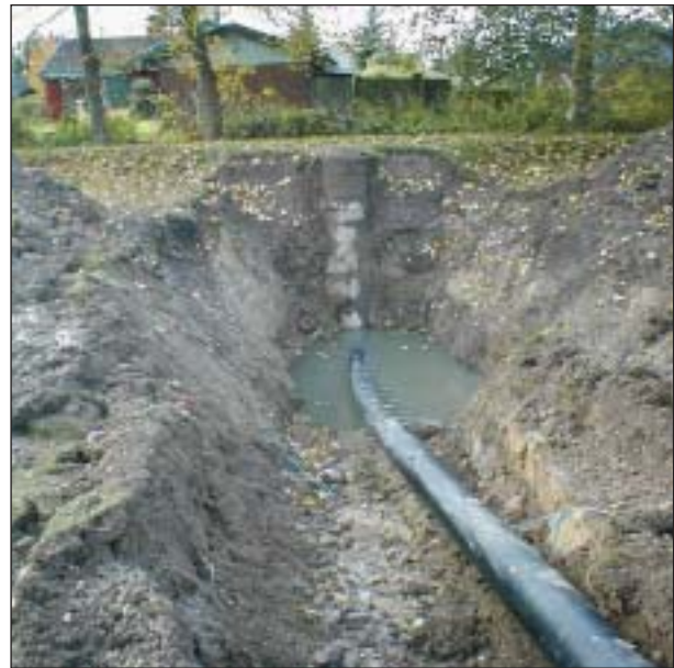
The control committee also inspects technical conditions, e.g. launch pit design.
